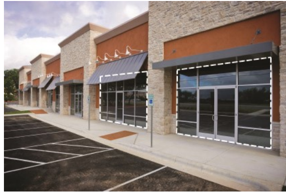
Figure 1119-H: The window area is illustrated within the dashed line area for the two storefronts in the above image. The dashed lines highlight two separate window areas due to the separation by an architectural feature not related to the windows.
