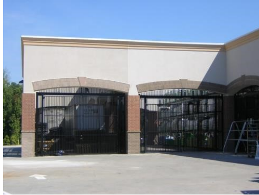
Figure 1115-C: Use of a wall and fencing for screening that is architecturally compatible with the principal building.
