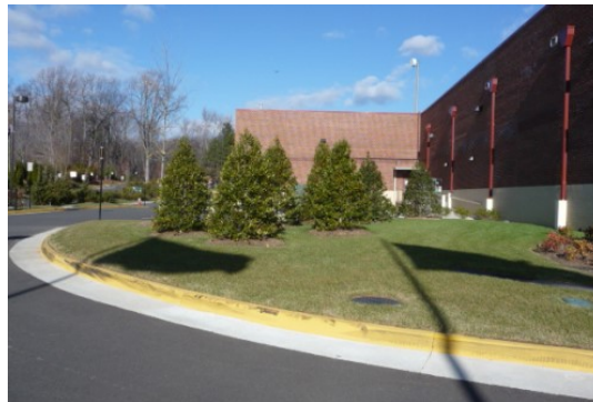
Figure 1115-D: The above image illustrates a vegetative screen that hides HVAC equipment and a dumpster.
