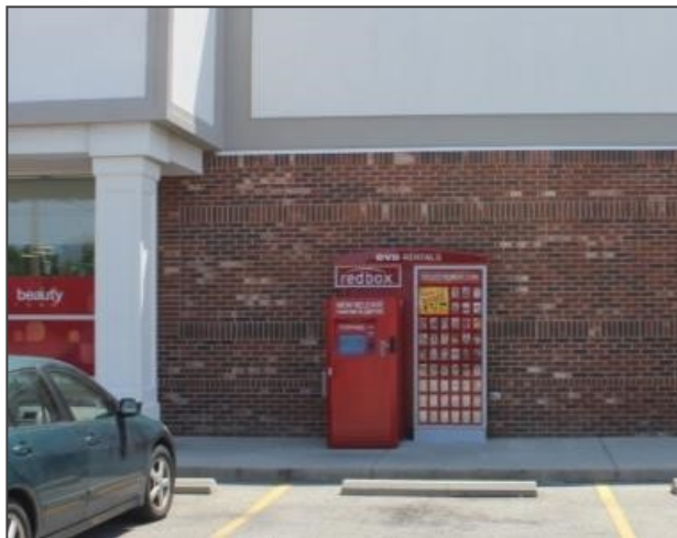
Figure 1111-A: The above is an image of a vending machine that is appropriately located along the façade of the building.
